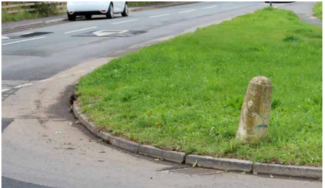
Kerb along B1228 opposite Elvington Primary School ▼
